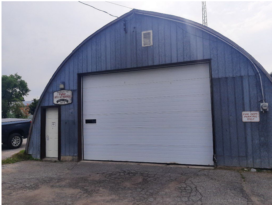
Photo 1 – Exterior view of the building.
